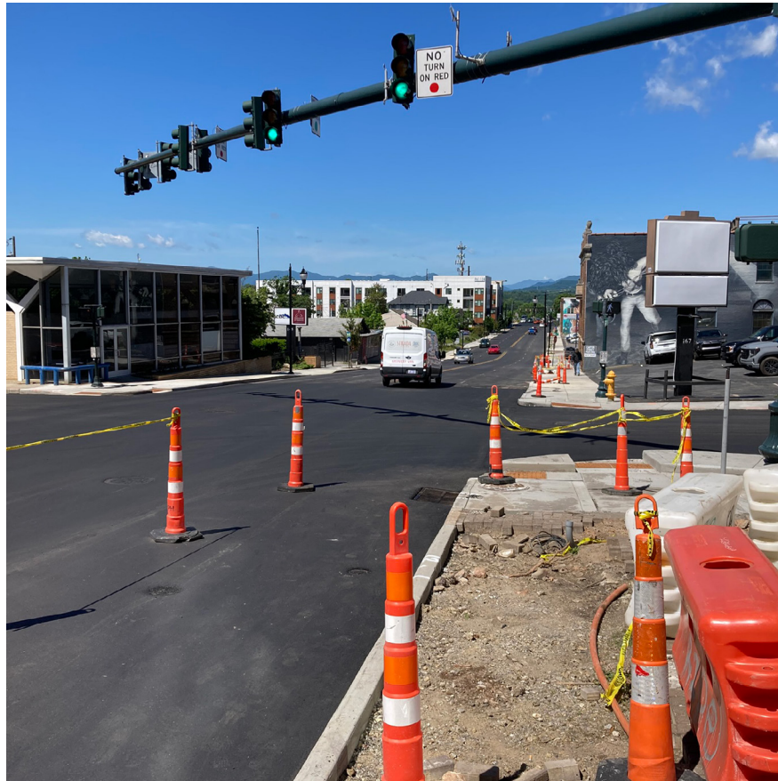
Image 8.1: Patton Avenue Construction (Looking West at French Broad Avenue)
