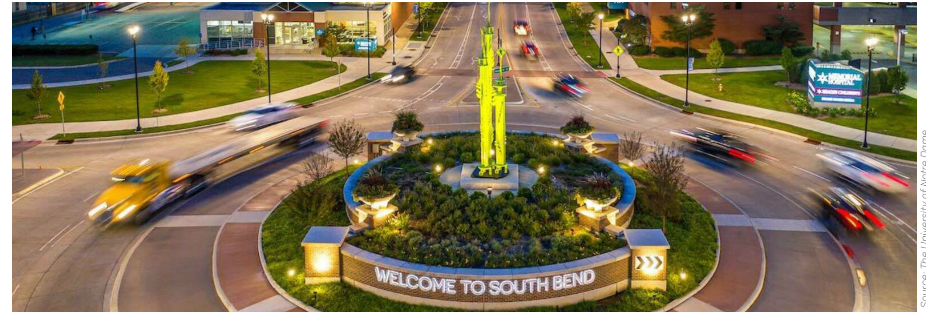
Image 6.1: Example of a Roundabout as Gateway Sign and Sculpture
