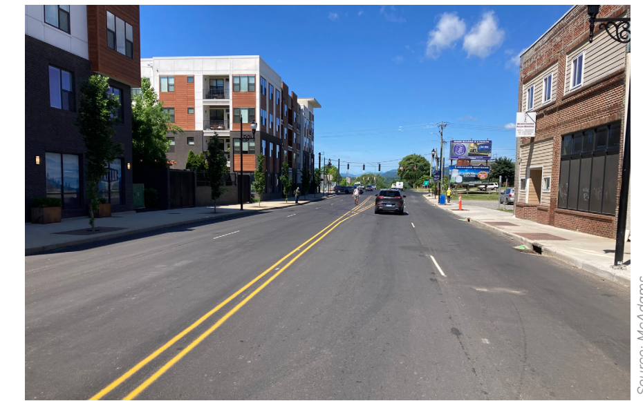
Image 2.2: Patton Avenue (Looking West from Pearl Street)
