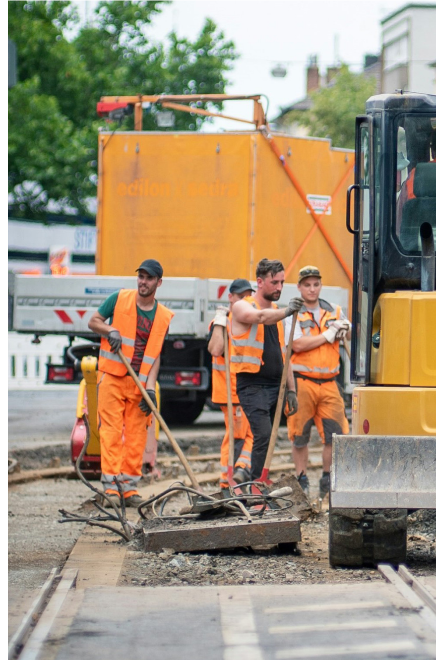
Image 7.3: Carter Ann Patton Stormwater Project Construction
