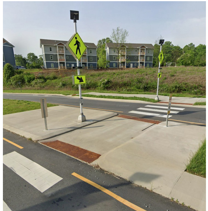
Image 6.5: RRFB on the Ecusta Bypass Roundabout in Brevard
